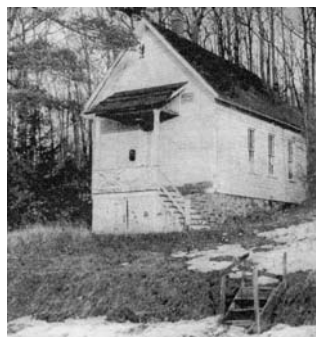
Fuller Hollow School District #15 on Powderhouse Road.
